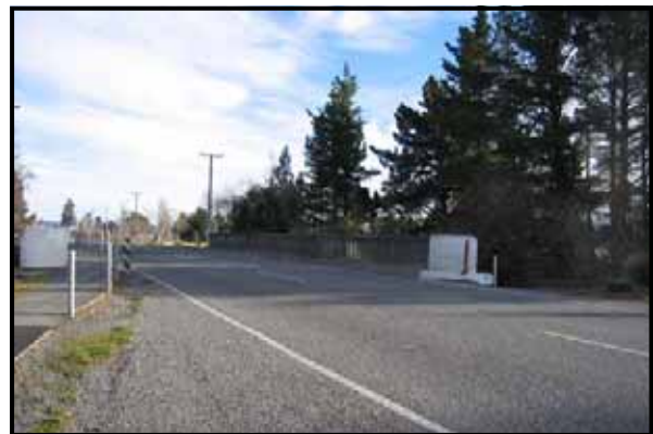
Bridge on northern side
